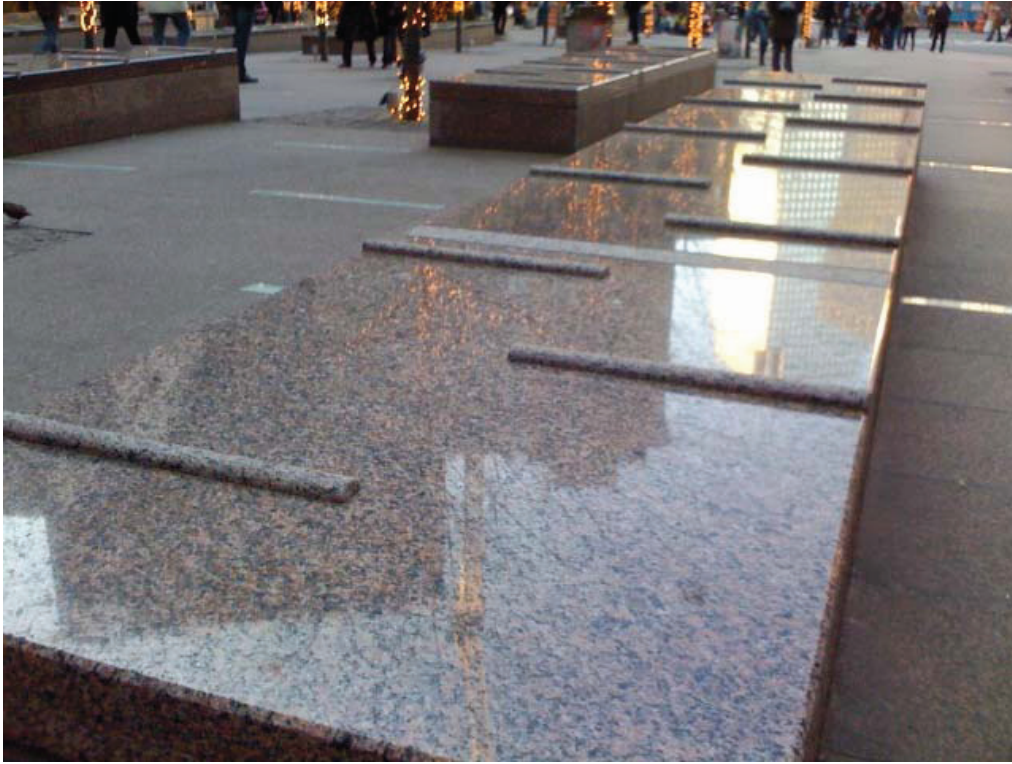
Figure 15. Anti-skateboard ridges embedded in the design of benches in Zuccotti Park, a public square in the Financial District of Manhattan. (Source: Author's Collection, 2008).
